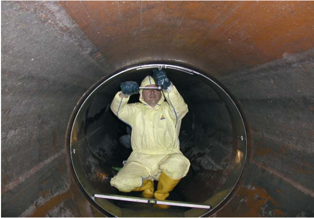
Positioning of sleeve
