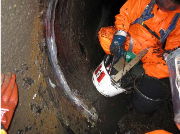
Remove sediments, equalizing offset with grouting
